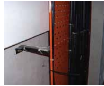
Figure 5.14: Vertical pipe installation on cable tray
